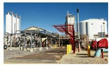
Small natural gas liquefaction systems produce up to 800 metric tpd (42 MMSCFD, or 0.3 MTA) of LNG for requirements such as peak shaving, transportation fuel, virtual pipelines or boil-off gas reliquefaction. Low cost and readily available refrigerants. Simple operation and superior turn-down efficiency. Modularized design minimizes construction costs.
